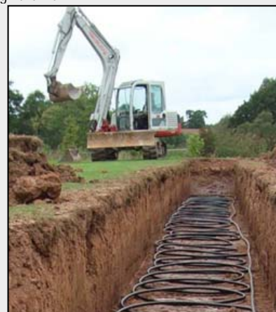
Installing horizontal ground loops (Source: Kensa Engineering)
